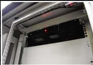
The CMC III monitoring system for monitoring the statuses in the safe
