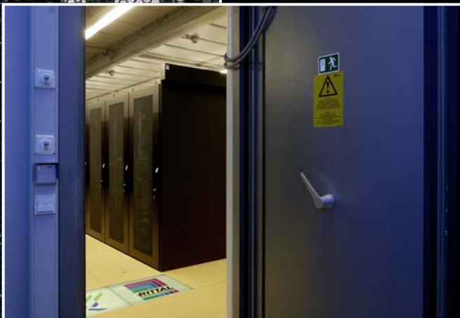
Security door of the ECB-S-certified High-Availability room
