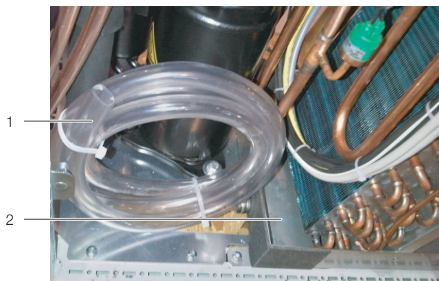
Fig. 23: Condensate discharge
