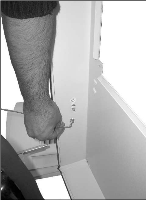
Fig. 77: Disconnect the earthing cable (2)
