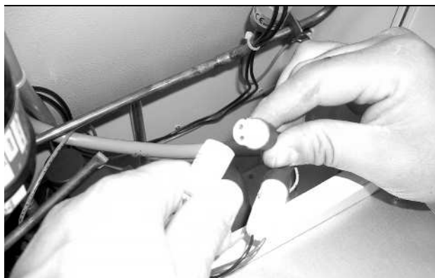
Fig. 71: Disconnect the fan connectors (3)
