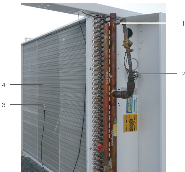
Fig. 32: Connection of sensors
