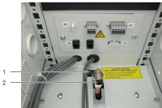
Fig. 53: Bleeding the air from the heat exchanger
