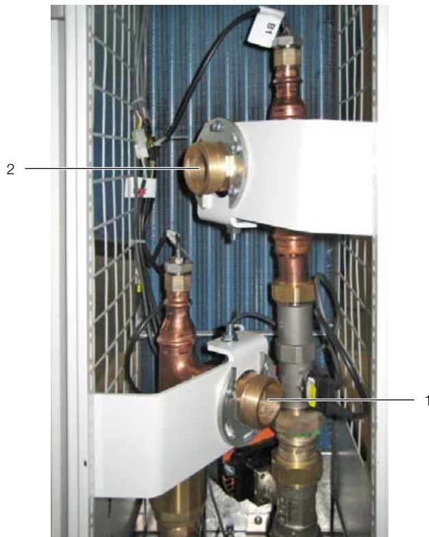
Fig. 46: Cold water network connection:
