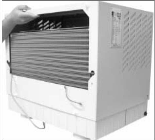
Fig. 37: Remove the cover
