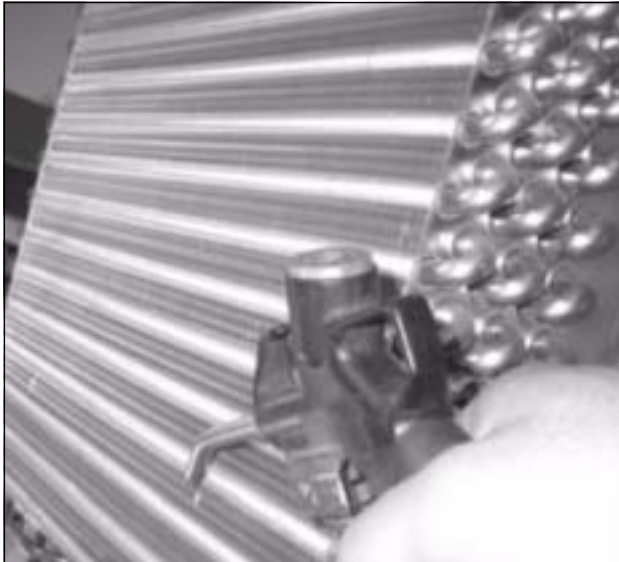
Fig. 40: Clean out the heat exchanger coil and compressor chamber using compressed air
