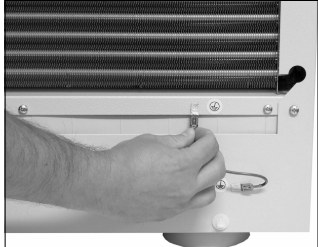
Fig. 27: Disconnect the earthing cable
