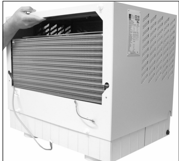
Fig. 29: Remove the cover
