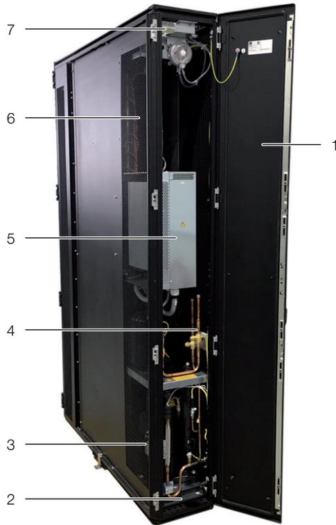
Fig. 8: LCP Rack DX rear – rear door open
